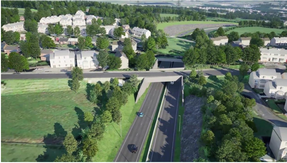
Caption: A new dual carriageway will run under a new bridge and underpass to the north of Mottram.
